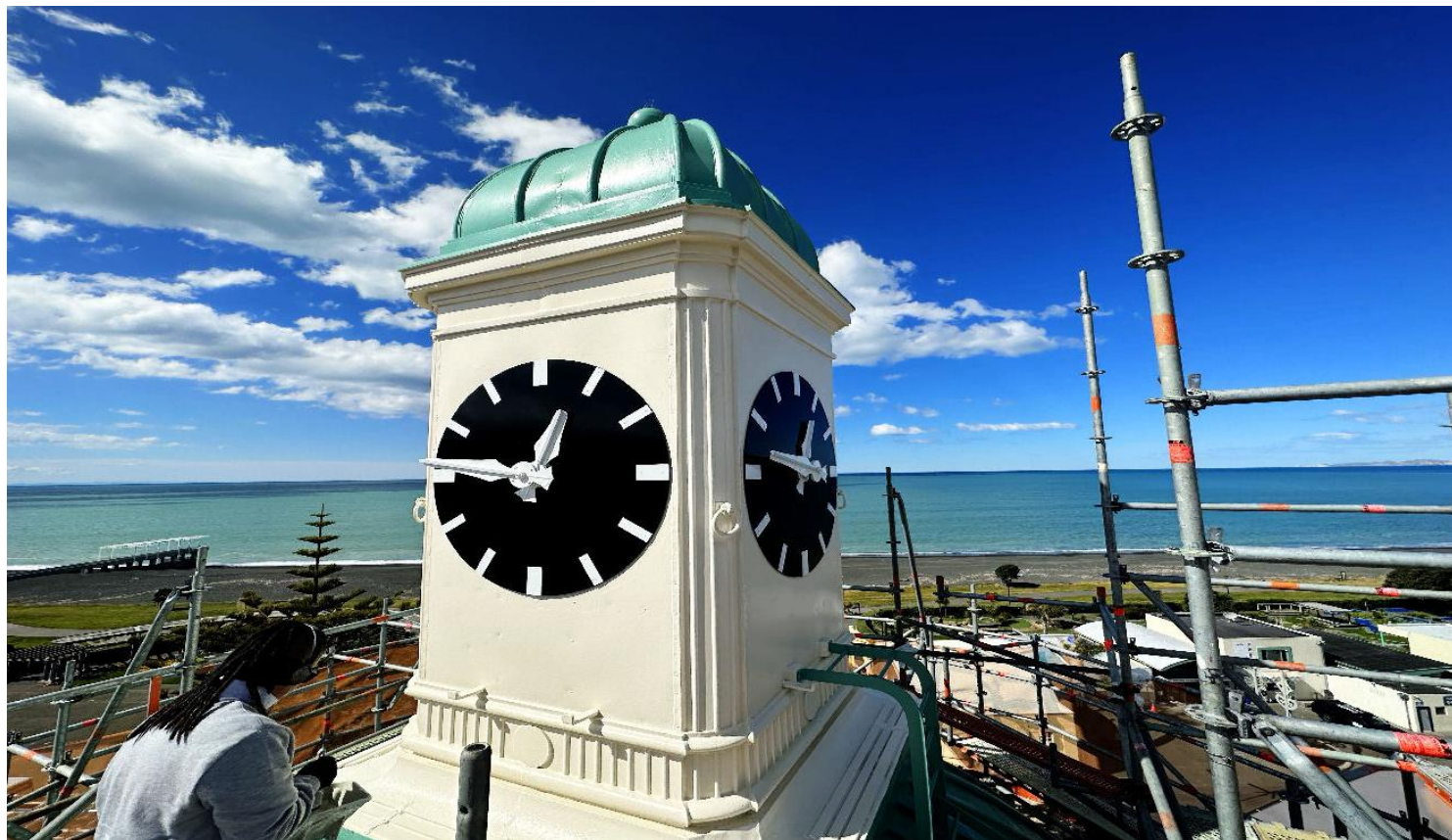
Scaffolding comes down from the T&G clocktower. Photo / Supplied
