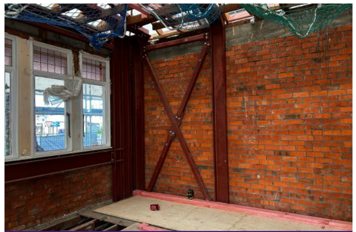
Seismic Strengthening since covered by lining. Photo / Supplied.
