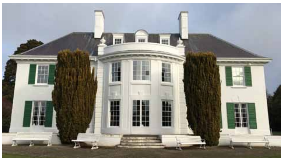
Anderson House, Invercargill – strengthened and upgraded.
