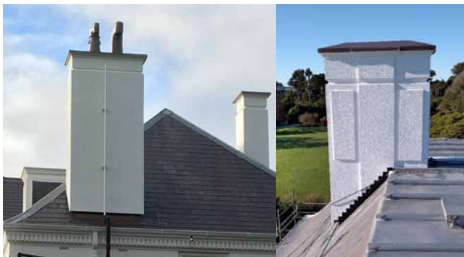
Chimneys were replicated in lightweight materials to reduce the risk of chimney collapse damage.
