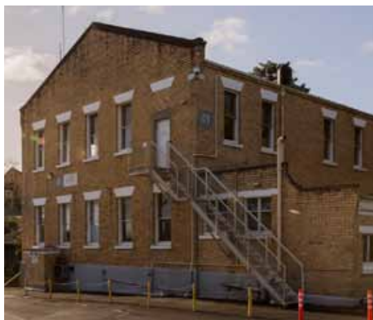
Building One's south wings, Carrington, Auckland.
