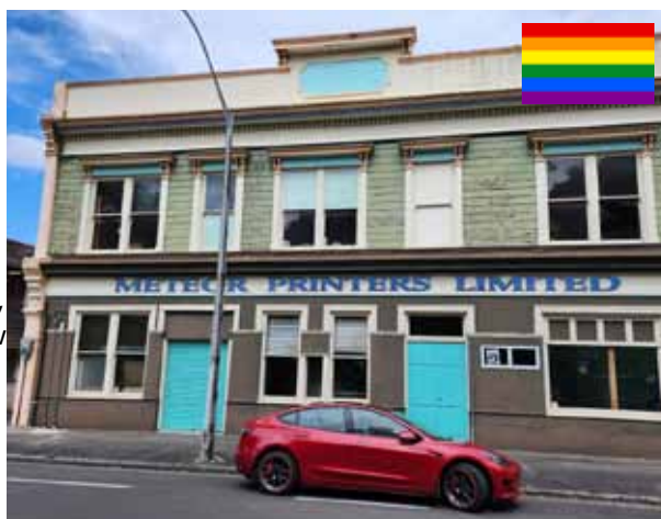
Duigan's Building, Whanganui. James Barron
