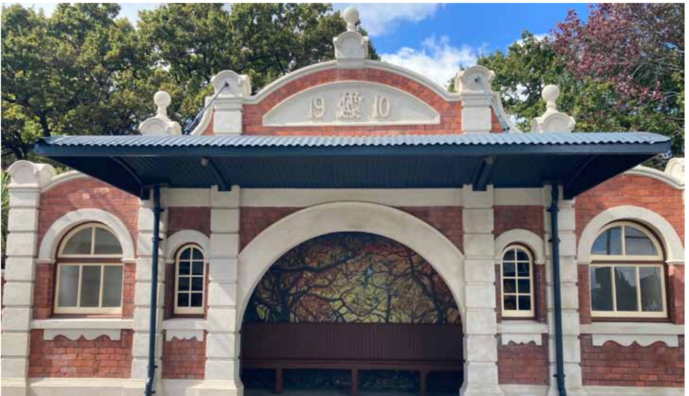
Symonds Street public toilets and tram shelter with interior view above, April 2022
