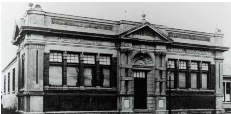
With the right vision, funding and people, Dannevirke's Carnegie Library building could remain.
