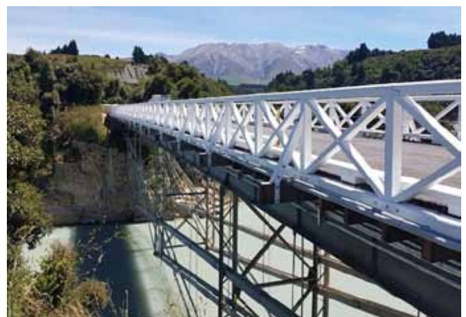
The repaired balustrade.
