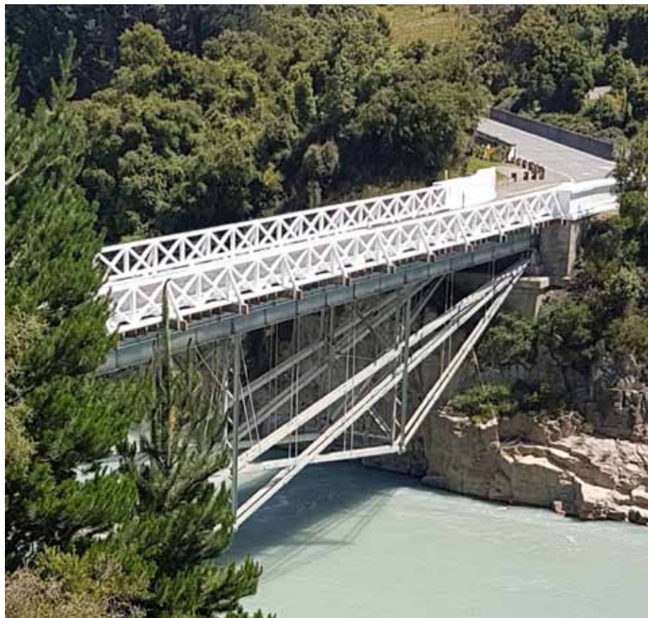
The Rakaia Gorge No.1 Bridge at completion of the project.
