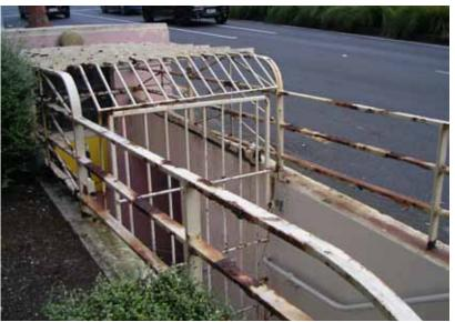
Wellesley St toilets before and (below) after rust was removed and the above-ground structure repainted.
