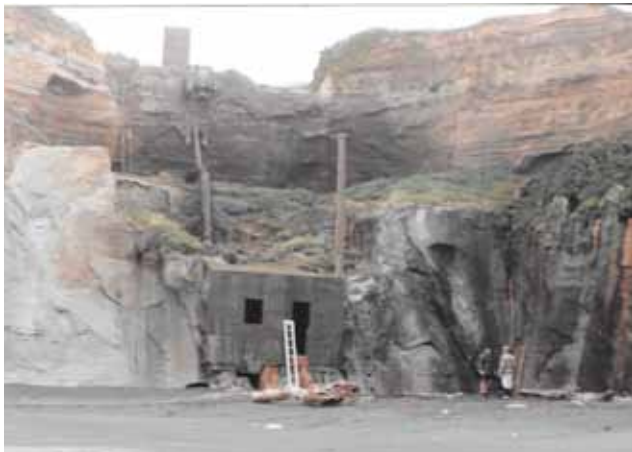
Patea Power Station c2010.
