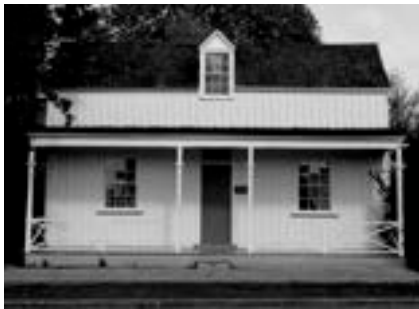
Wyllie Cottage, Gisborne, is an 1872 example of a building that uses balloon framing.
