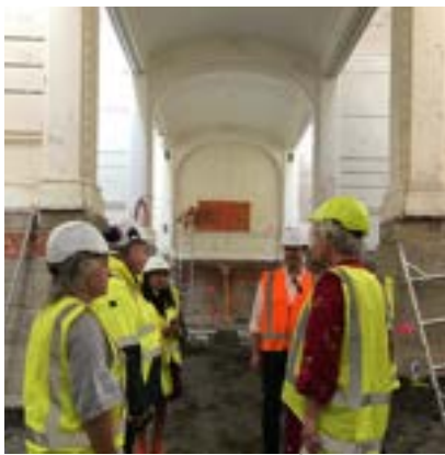
UNESCO commissioners view the Sarjeant Gallery building site.
