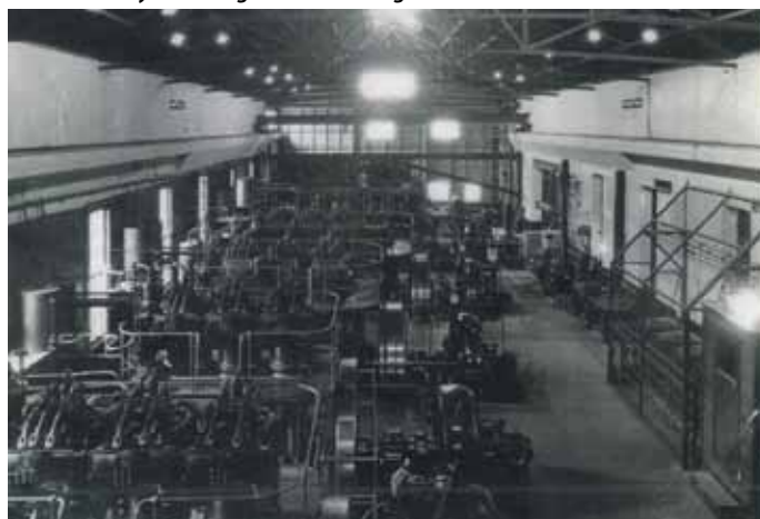
Hawke's Bay Electric Power Board building, Hastings, and (below) engine room after 1925 showing all six generating units in place with three cylinder engines in the foreground.
