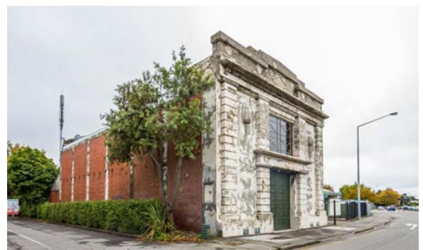
Milton Street Sub Station, Christchurch, being strengthened and redeveloped as a commercial property with EQUIP funding.
