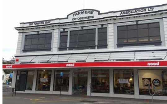
Mid City Plaza, Napier, strengthened with EQUIP funding
