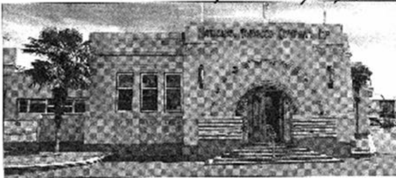
OPEN FOR SUMMER: The National Tobacco Company building in Ahuriri. PHOTO/SUPPLIED
