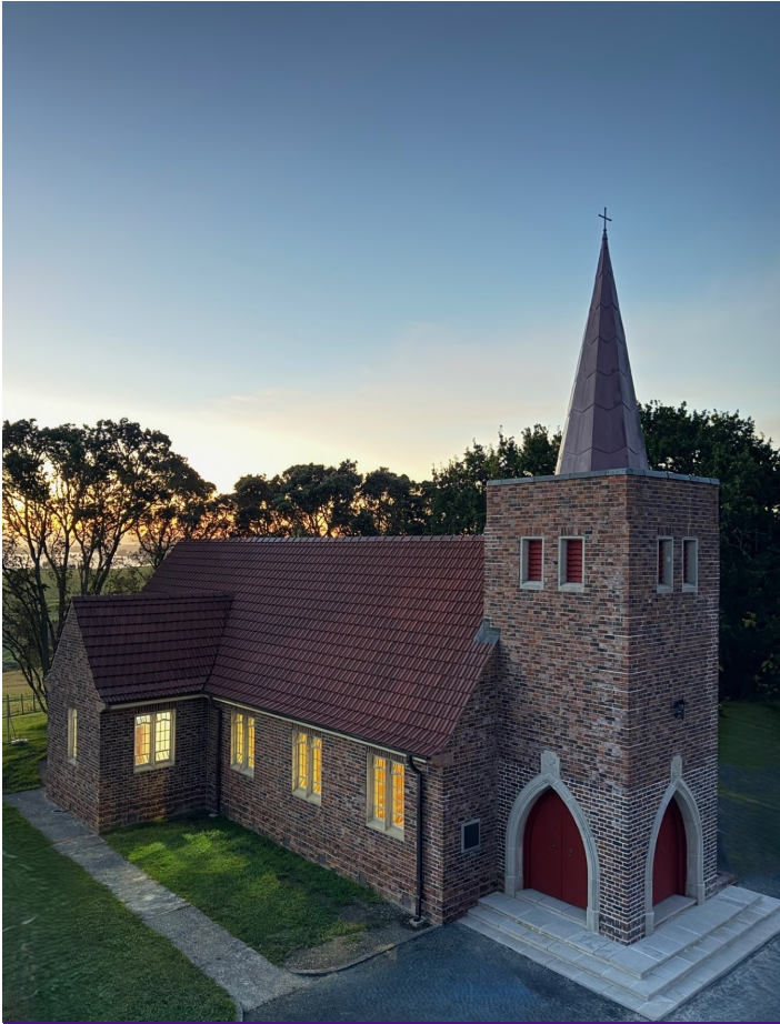
Restored exterior of Coates Memorial Church. Photo / Blake Morris, Argon Constructors Ltd
