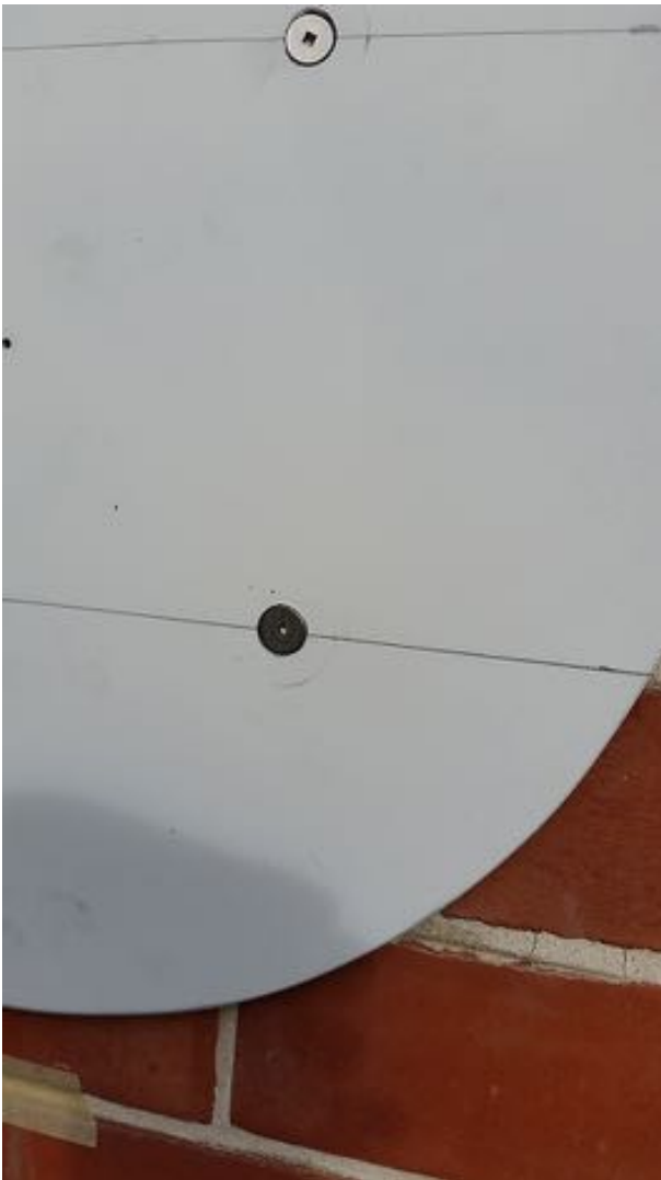
9) Insert each screw so it is flush with face of ACM backing plate
