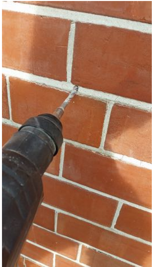
4) Drill holes in mortar joints
