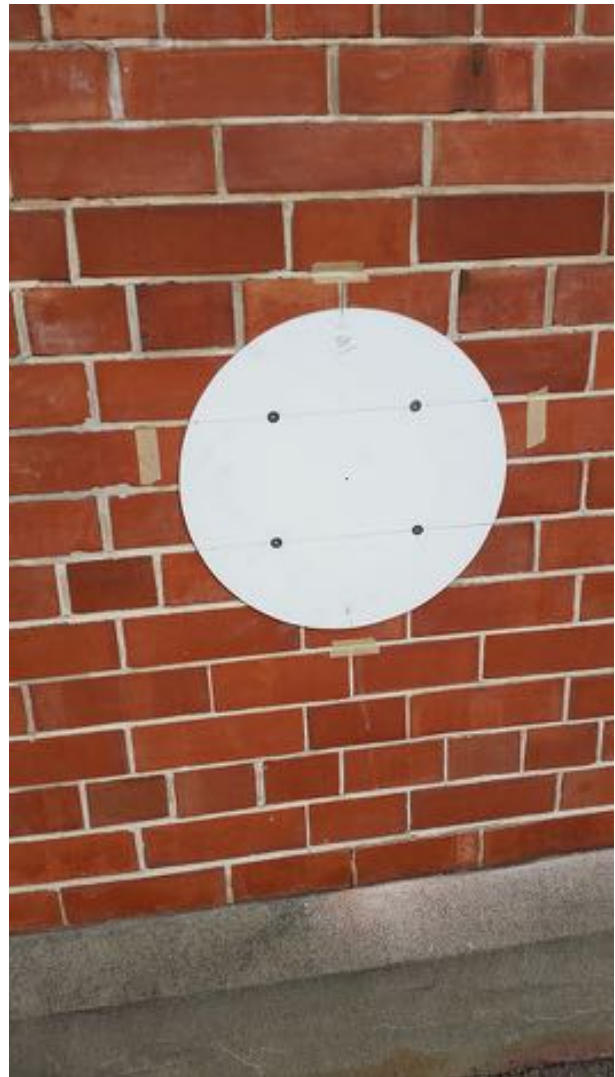
10) The backing plate secured into position
