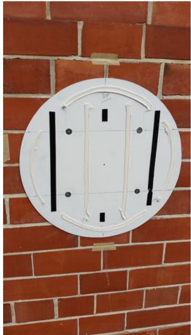
14) Peel off other side of protective strip from 3M Automotive Acrylic Plus Attachment Tape
