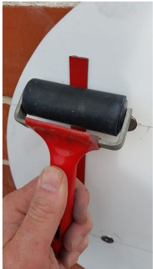
12) Peel one side of 3M Automotive Acrylic Plus Attachment Tape and place backing plate. Use a roller to ensure adequate adhesion
