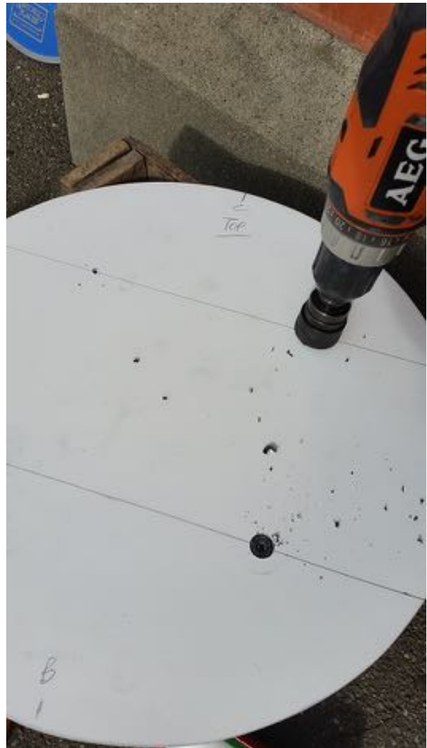
6) Drill recesses into aluminium signboard backing plate using ACM Drill Tool. This will ensure that the screw heads finish flush with the surface of the ACM backing plate
