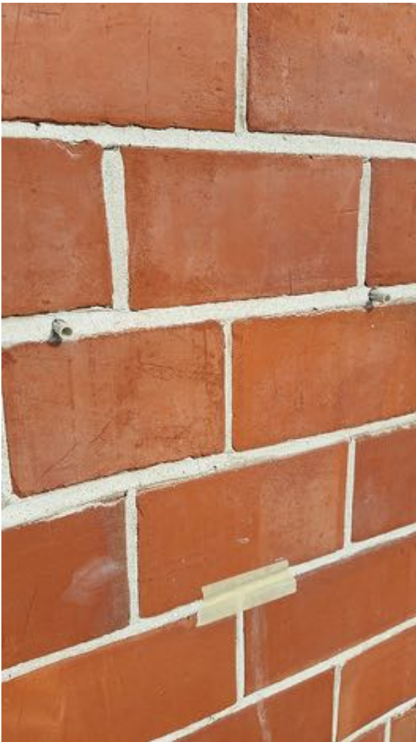
5) Insert plastic plugs into holes
