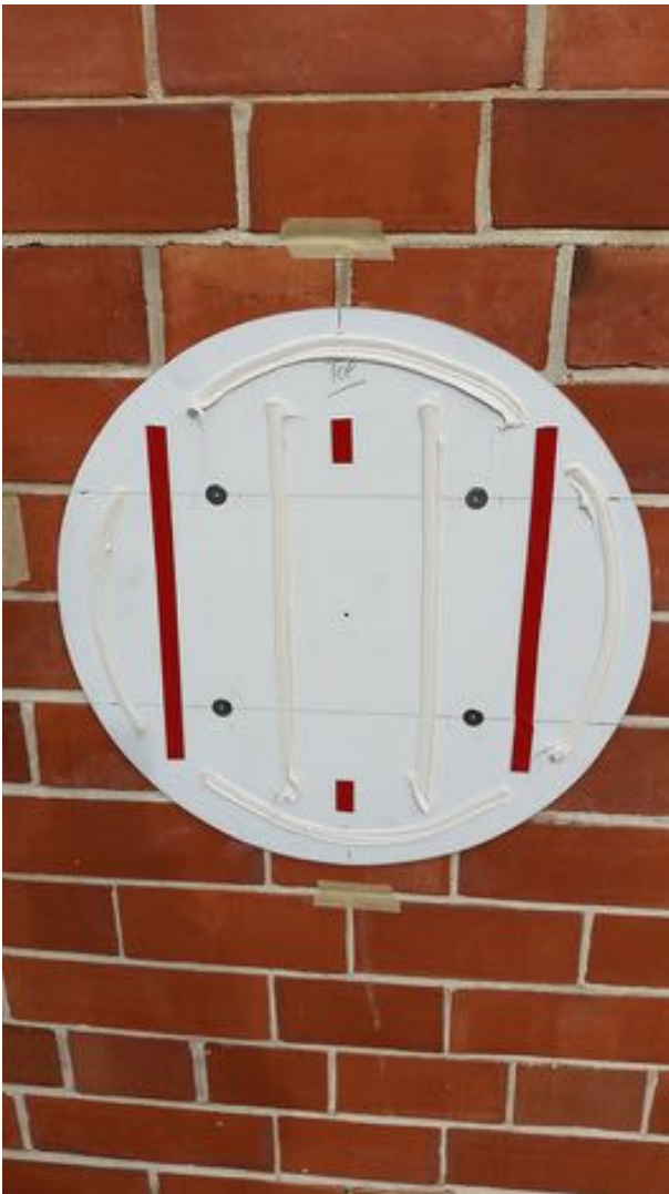
13) Apply 'Siroflex' Grip & Grab adhesive to the backing plate
