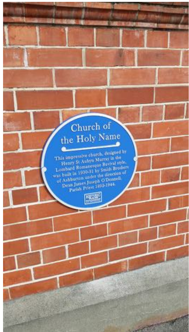
18) Once plaque is correctly positioned and secured in position, the masking tape can be removed
