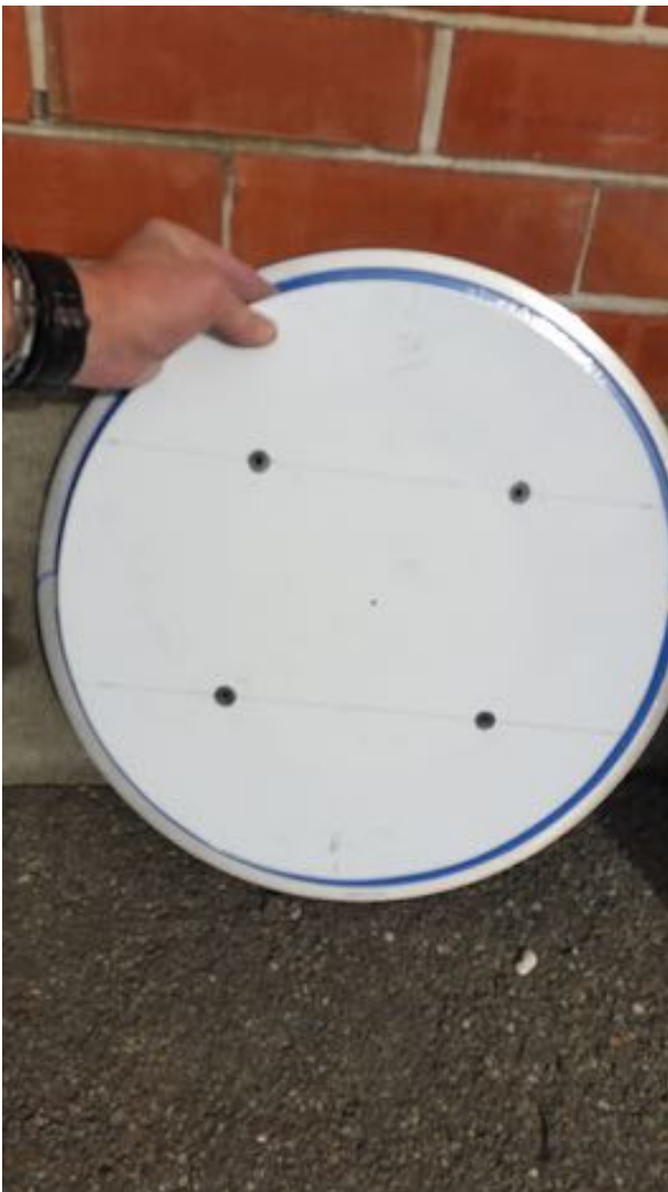
7) Note that circular aluminium 'signboard' (ACM) backing plate is cut smaller than the size of the blue plaque (400mm diameter)
