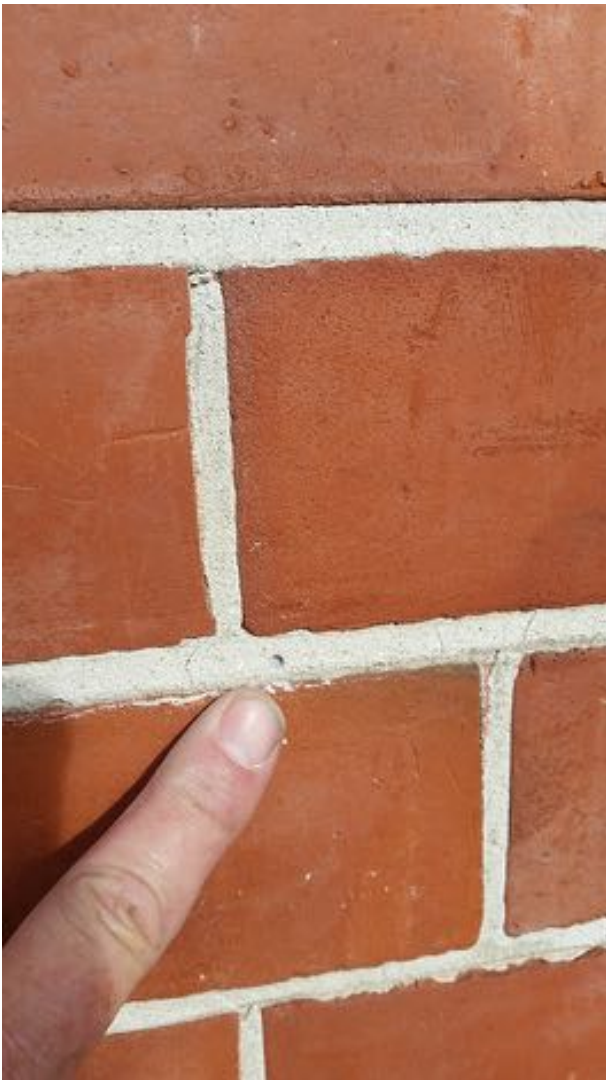
3) Mark pilot holes in mortar joints
