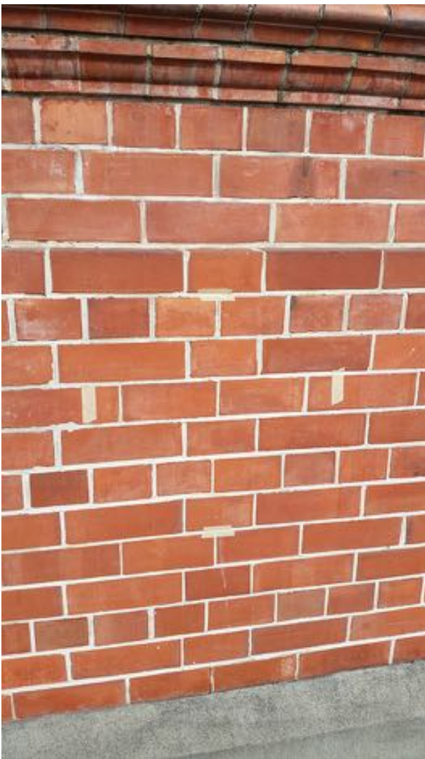
1) Mark-out the proposed position of plaque with masking tape
