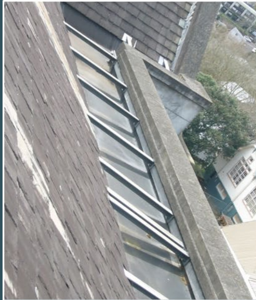
Structural steel fitted at flashing /upstands level
