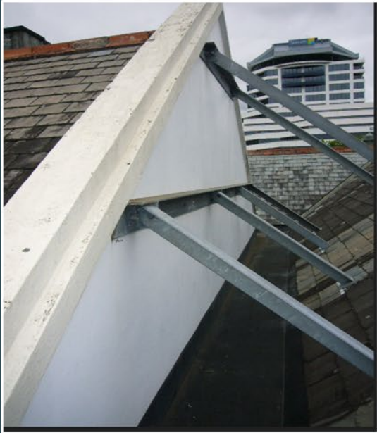
Steel restraints to gable walls
