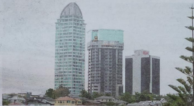
More tall apartment buildings are likely on Takapuna's future skyline.
