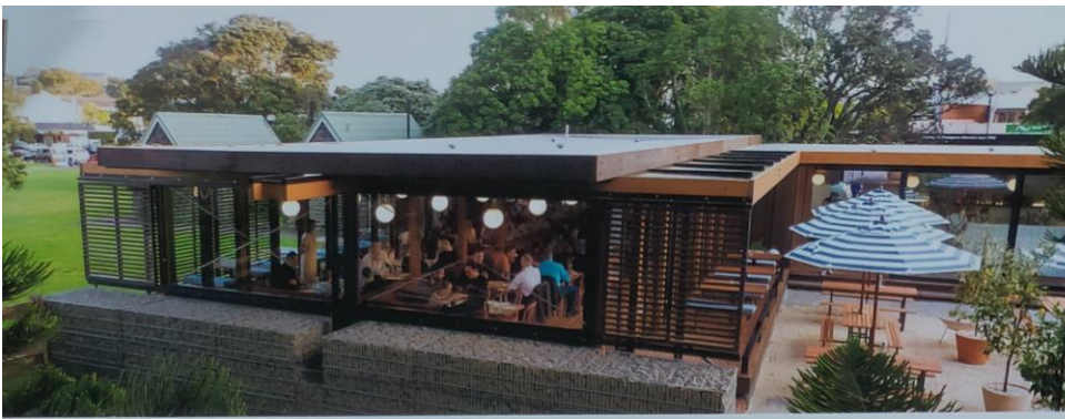
Melanesian Mission showing contemporary additions giving the heritage building new life as a café and restaurant.
